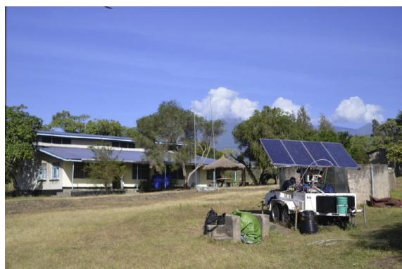
Fig. 7. Photo of the solar-powered hybrid UF-NF/RO system at the NDRS to where Site 4 water was transported for experiments.
