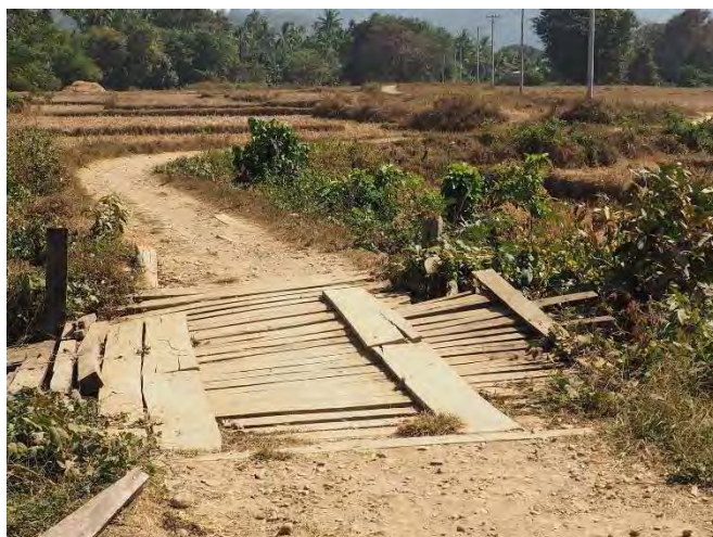
FIGURE 22: THE BRIDGE ALONG THE SOE BON VILLAGE MAIN ROAD
