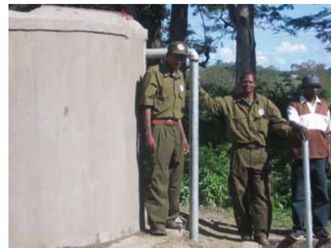
A total of 85 km of gravity water pipe systems was constructed. The system collects water from 6 springs and 2 deep wells and brings it to 15 reservoirs storing 755 m 3 .
